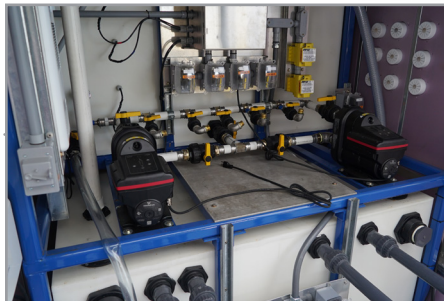
Interior View of Trailer
