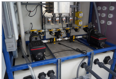
Interior View of Trailer
