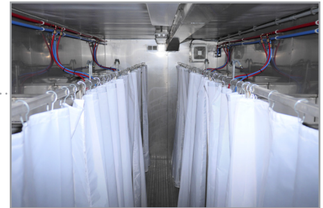
View of the shower area
