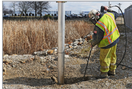
A technician using pressurized water to dig
