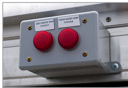
Freshwater and greywater capacity indicator lights.
