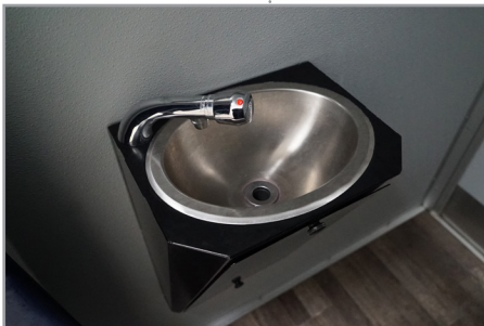
View of sink
