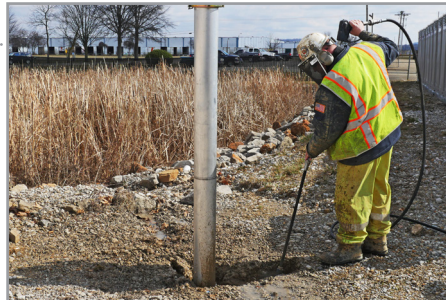
A technician using pressurized water to dig
