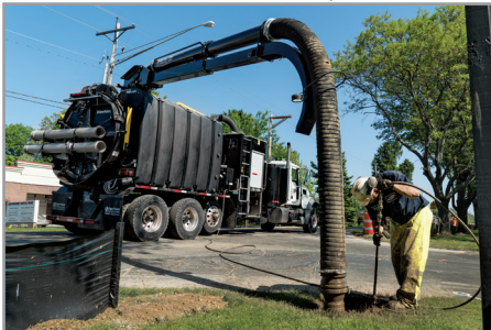
Porta Kleen's Hydro-Excavation truck on-site
