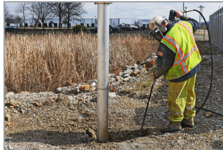
A technician using pressurized water to dig
