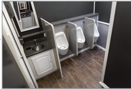
Interior view of urinals and sinks
