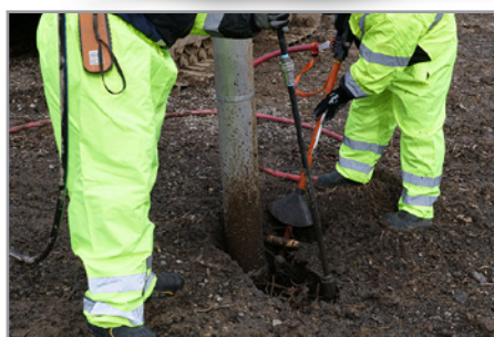
Dig simultaneously with water & air
