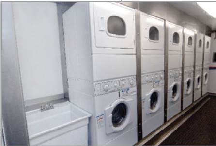
View of the sink, washers, and dryers
